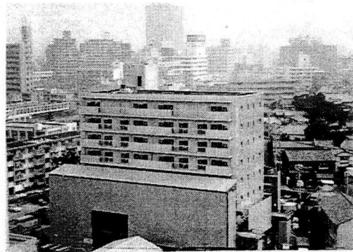
Photo 4: Exterior of Building During Construction
