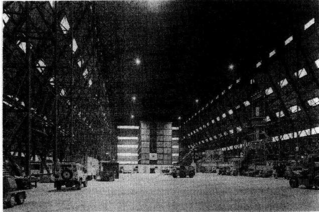
The Cardington Laboratory - 8-storey building at rear
