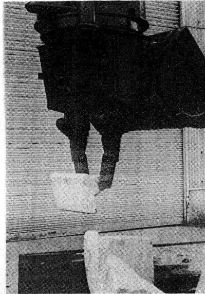
Photo.-2 The scene of holding a prefabricated concrete block
