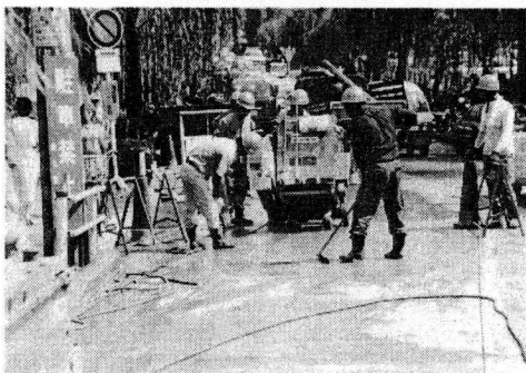
Photo 1 Conventional cutting work(1)
