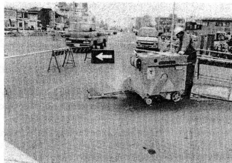
Photo 2 Conventional cutting work(2)
