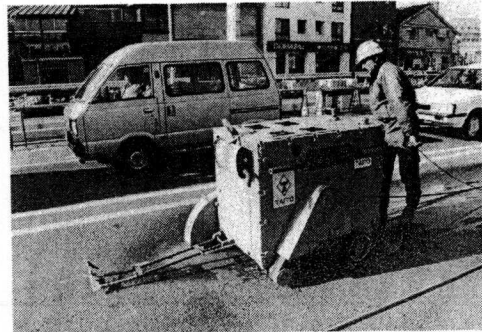
Photo 3 Conventional cutting work(3)
