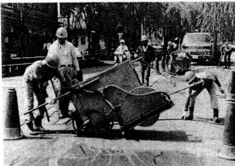
Photo 4 Conventional cutting work(4)
