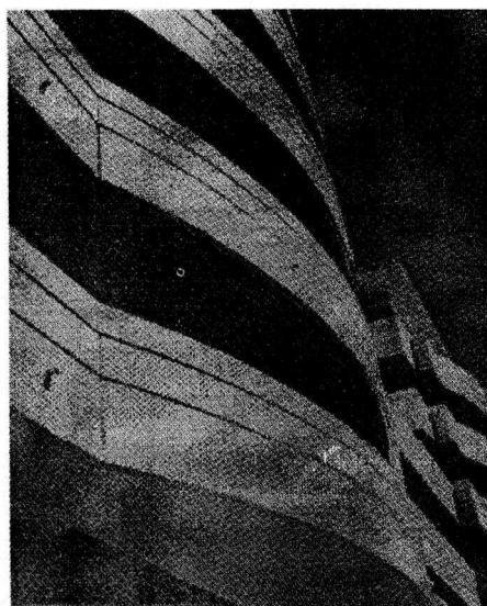
Fig. 1 Typical facade using GRC panels
