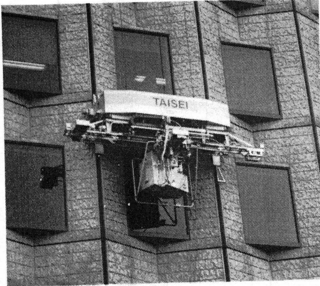
Photo 1 Robot for painting exterior walls
