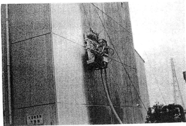
Photo 3 Painting of the Struc- tural Concrete Wall by the Painting Robot
