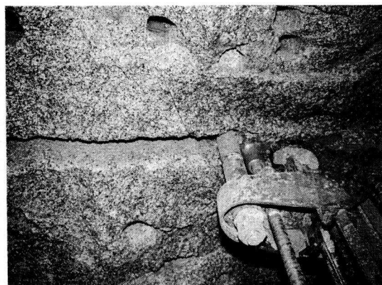
Figure 4. Continuous hole drilling
