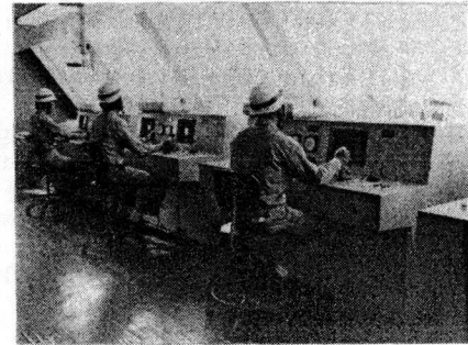
Photo.4 Operating Room in the Execution Ship
