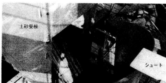
Photo 2 Soil receiving board and chute
