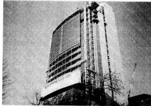
Photo 4. Situation of the automated exterior curtain wall installation system.
