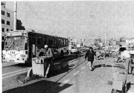
Photo 1 Pavement cutting work
