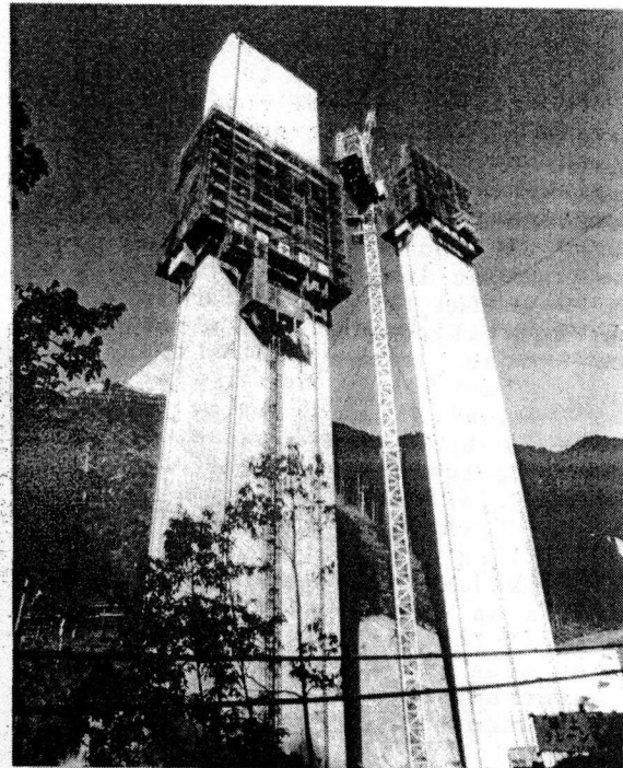
photo-2 State of construction
