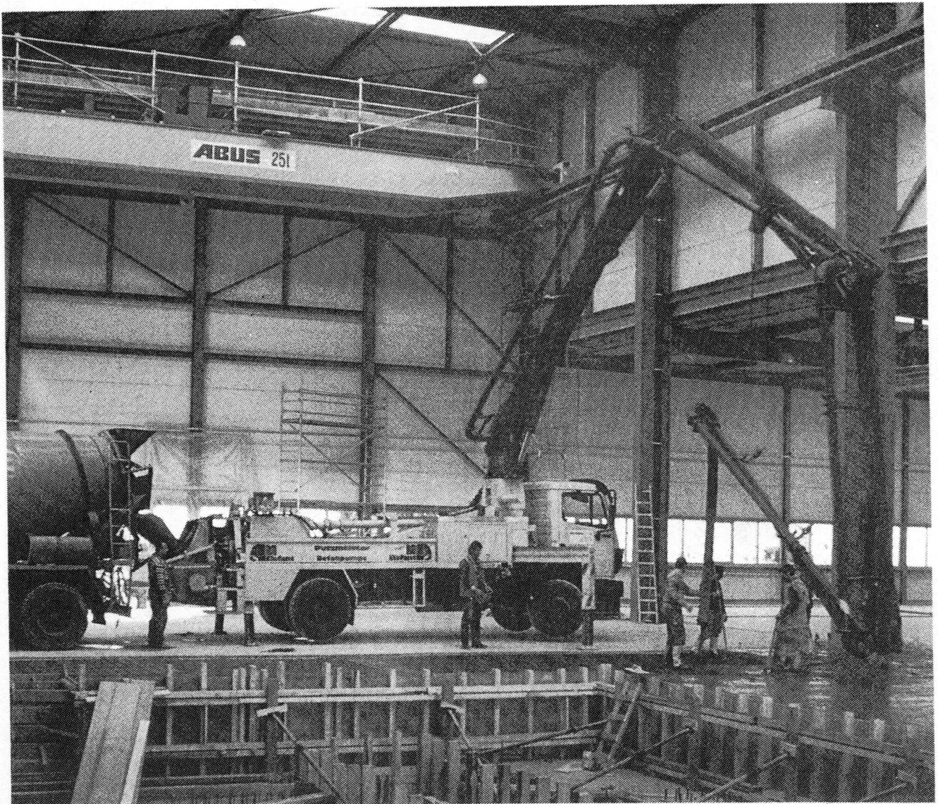
Fig. 9 Computer aided concrete pump with 24 m 4-section boom in operation
