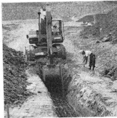
(2) Excavating and Finishing
