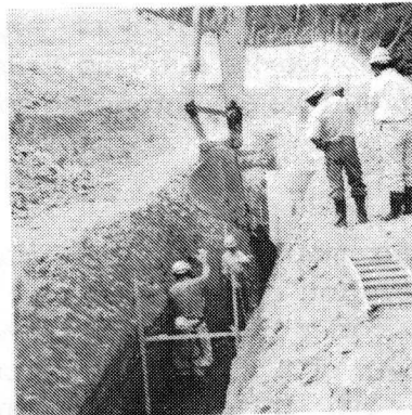
(3) Placing Crushed Stones
