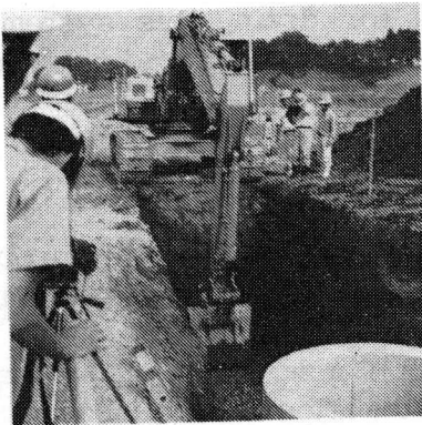
(3) Placing Crushed Stones
