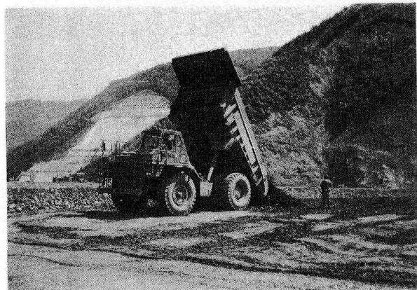
Photo.4 State of Laying
