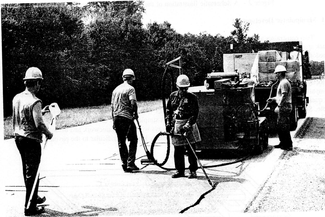
CRACK SEALING AT A TEST SITE ON ROUTE 90
