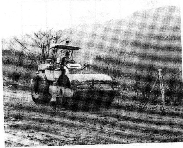
Photograph 2 Travelling Test Using Vibratory Roller
