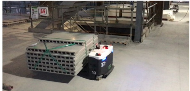
Figure 7. Trial at construction site
