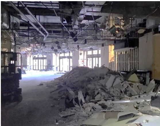
Figure 1. Active demolition project
