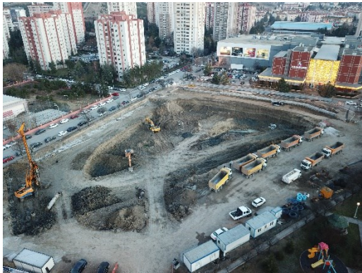
Figure 2. Aerial View of Construction Site at T1 Site Visit
