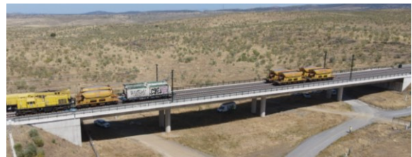
Figure 1. Viaduct La Plata during the load test
