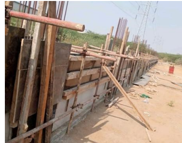
Figure 7. A retaining wall under construction with an unclear project type
