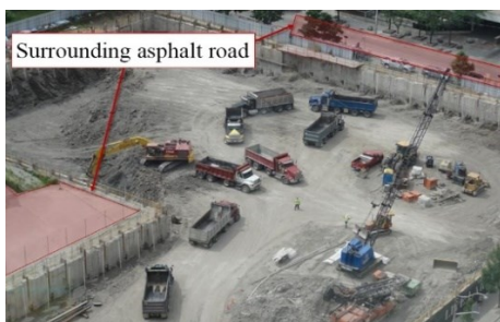
Figure 6. Asphalt roads beside a building sub-structure project
