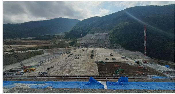
Figure 3. Overlook of autonomous construction of Naruse Dam in Japan.[20]
