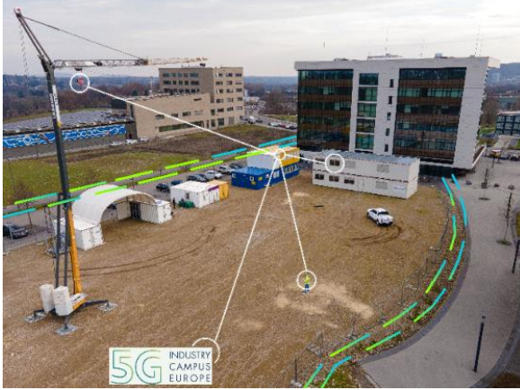
Figure 1. Construction Site operated by Center Construction Robotics in Aachen.
