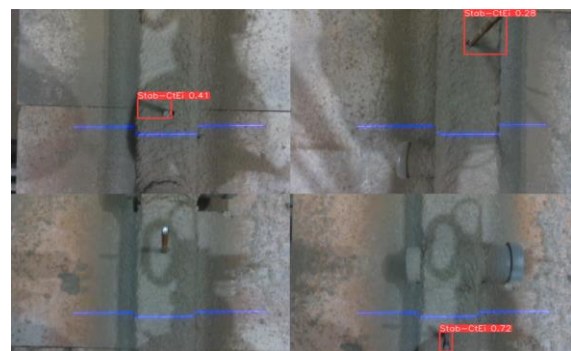
Figure 10. Images recorded during SC3DP evaluated by the trained CNN to label the inserted short rebars.
